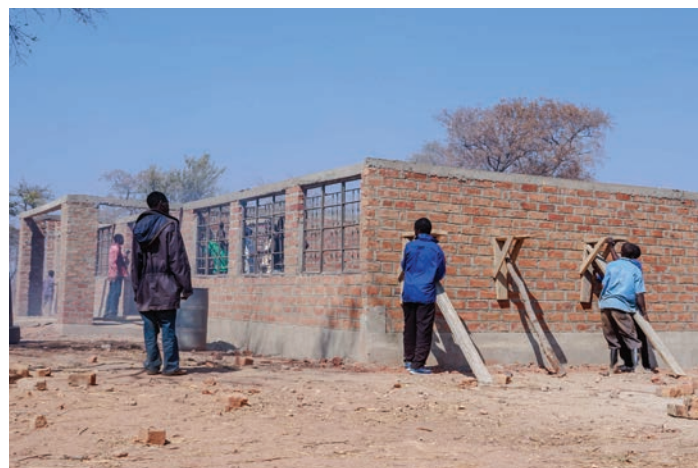
Work in progress at the school, Photo by Bellah Zulu, Zimba, 2016
