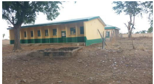
Below: Renovated laboratory at Yakawada Secondary School in Giwa LGA of Kaduna
