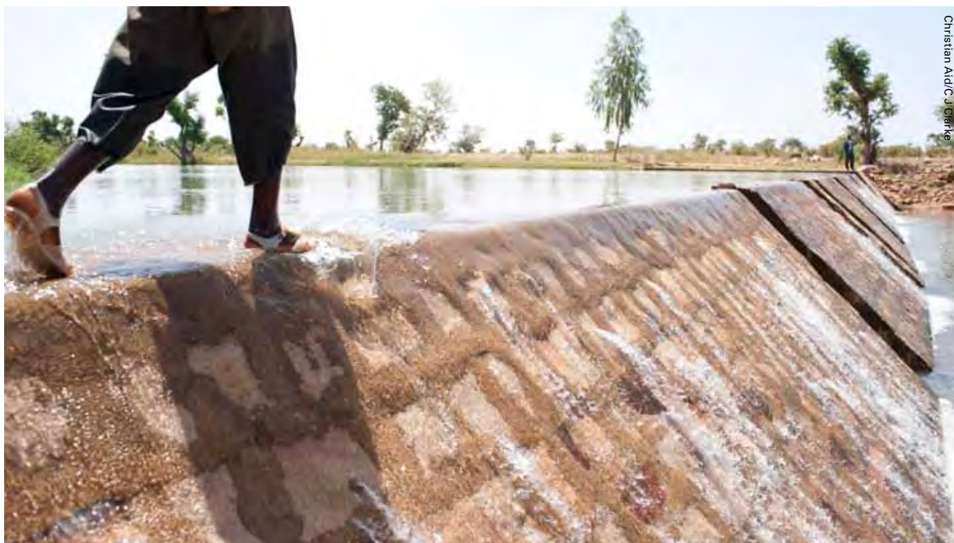
In Yowakanda village, Mali, a dam built with the assistance of Christian Aid partner APH Bandiagra helps the villagers to conserve what precious little rainfall they can in order to water their crops
