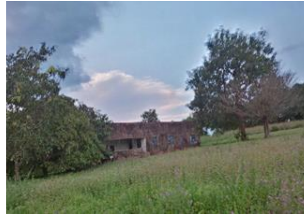
Below: The PHC in Alifeti that is supposed to serve the neighbouring communities including Ojuwo-Ojekele.
