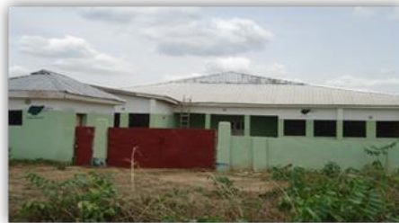
Below: The HP in EGBA that hasn't been commissioned and is not in use
