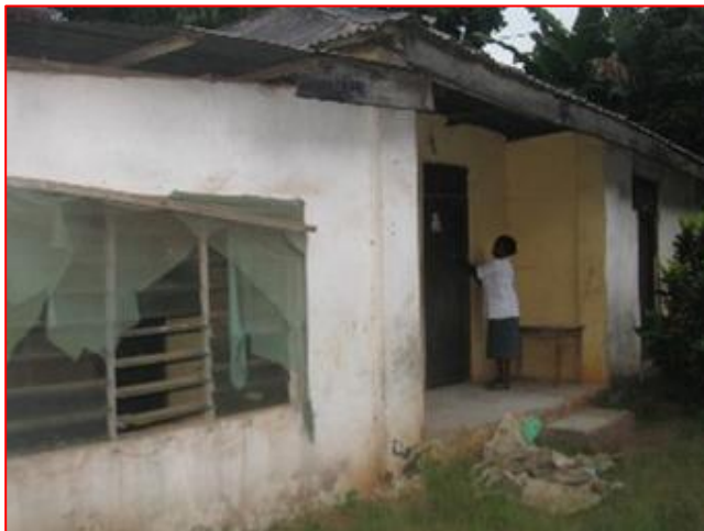
Below: Staff Quarters-PHC Oye Achina
