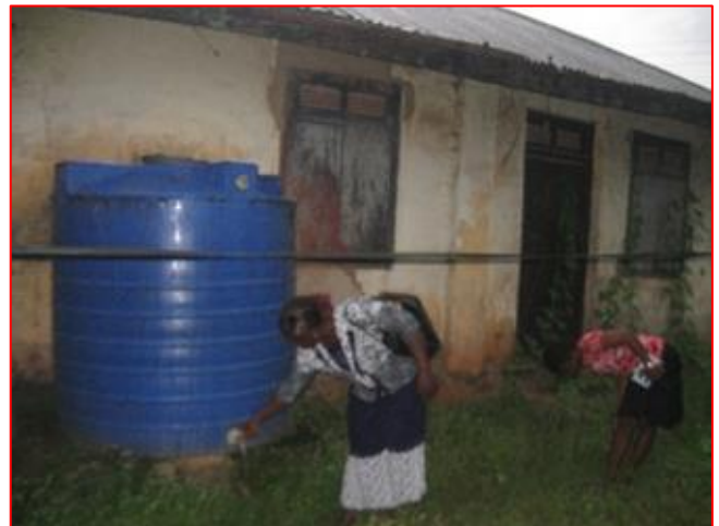
Below: Similar system of water supply across the PHCs
