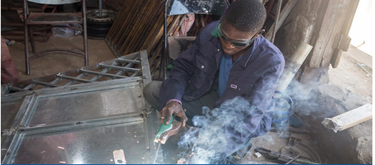
Shaifu Abdul Razak welding a metal door at his workshop in Nima Down Side. Shaifu has learned new skills through the GEOP programme, increased his income and is looking to take on and train more apprentices.
